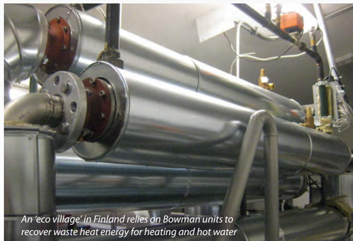
In Canada, Bowman exhaust gas units within a Cogen system, provide heat for a remote 'off-grid' community
