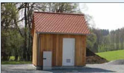
Example: Installation in a Machine house
